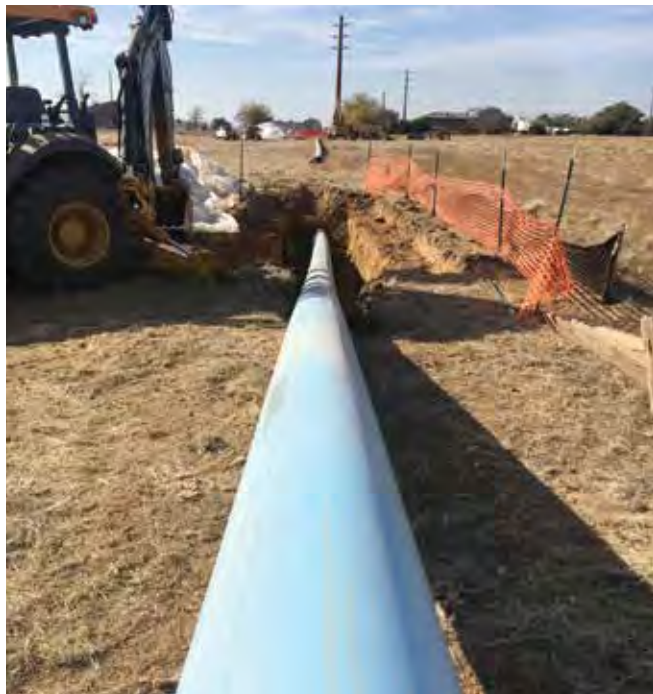
Pipe was installed in typical run lengths of 500-1,000 feet
