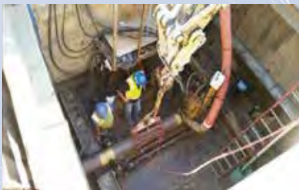
Front Steer Guided Boring, Drill Casings Installation
