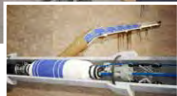
Lateral can be lined in one step with a remotely operated inflatable packer
