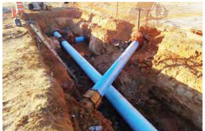
Fusible PVC® pipe utilizes standard waterworks fittings for reconnections
