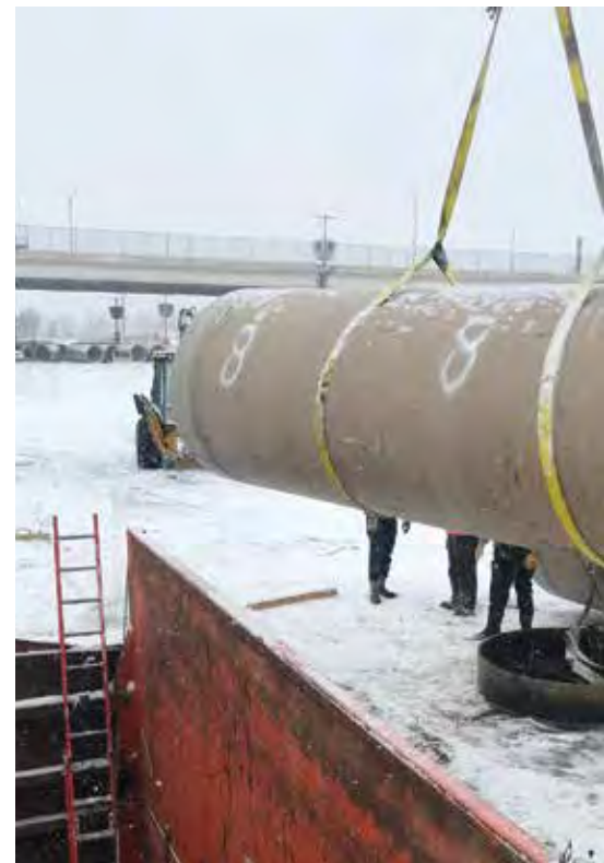
Twenty-foot pipe segments were lowered into the insertion pit
