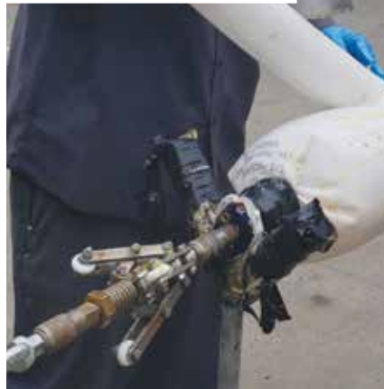
Lateral can be lined in one step with a remotely operated inflatable packer
