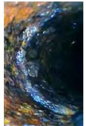
Cast iron corrosion
