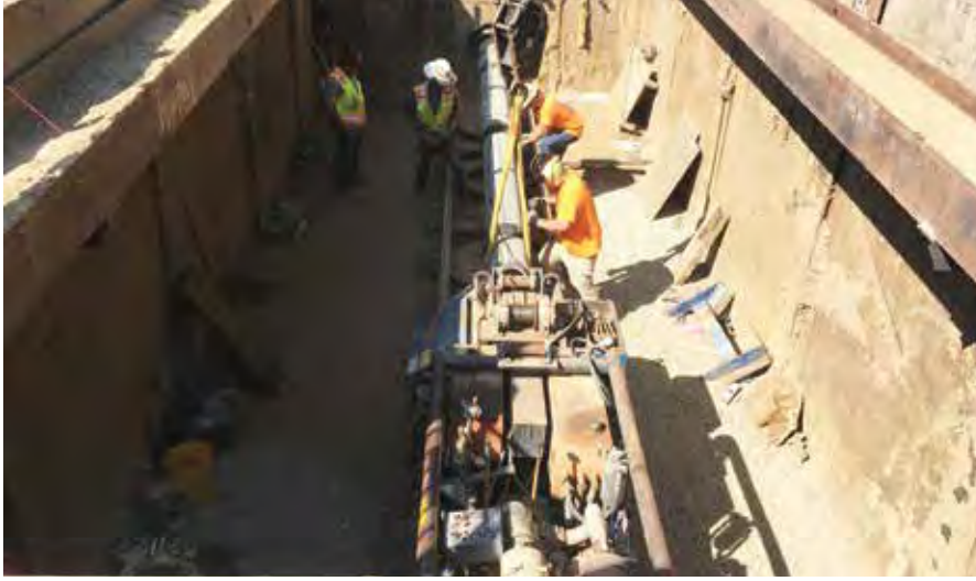
Figure 7. Installation of 12-inch cement-mortar lined and coated steel carrier pipe inside the 20-inch casing installed with guided boring took three days.
