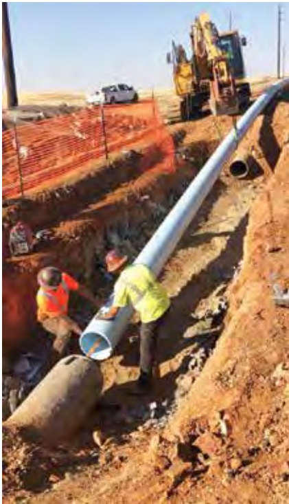
Pipe was pulled using the winch cable, which worked well
