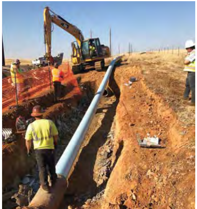
Fusible PVC® pipe during the slipline insertion process
