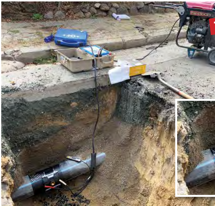
Typical Electrofusion Joint
