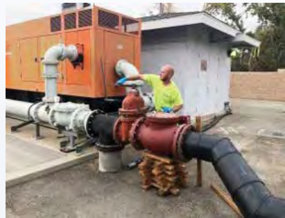
Bypass pumping for CIPP Project
