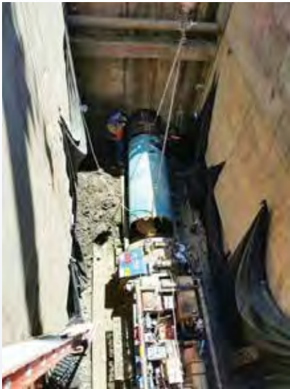
Pilot Tube Guided Auger Boring, 36-inch I.D. Steel Casing
