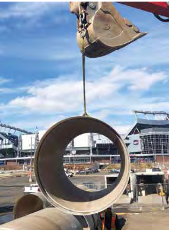
Ten-foot pipe segments were used to slipline the curved section of host pipe
