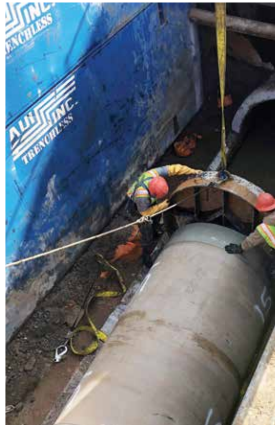
Custom fabricated push plate was used to evenly push the pipe into the host RCP using an excavator
