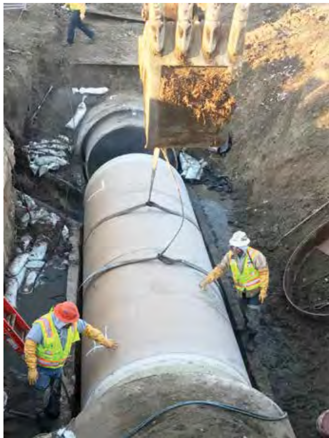
Sliplining 84-inch pipe inside the 90-inch RCP set a new record for the AUI crew!
