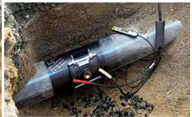
Typical Electrofusion Joint
