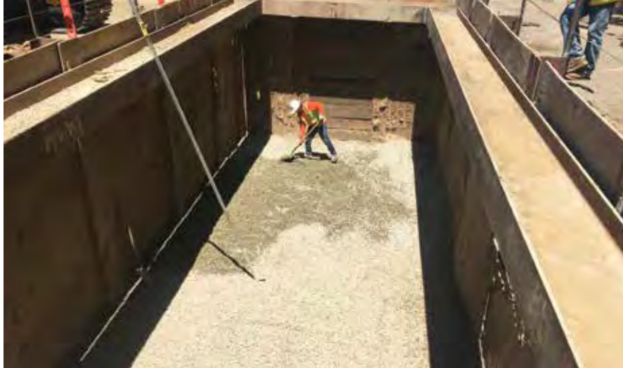
Figure 2. Launch shaft constructed using soldier piles with steel plate lagging due to low groundwater and stable ground conditions.
