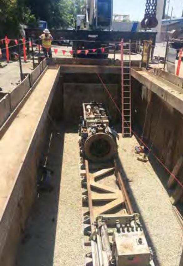
Figure 3. Auger boring rig set in the launch shaft with pilot tube guided boring equipment in foreground. Installation of 250 feet of guided pilot tubes took two hours.
