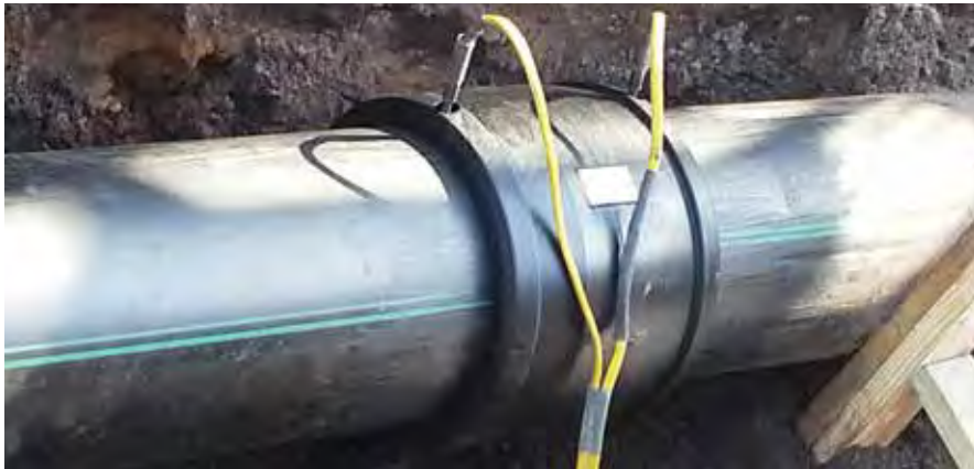
Electrofusion has proven to be an extremely reliable joining system
