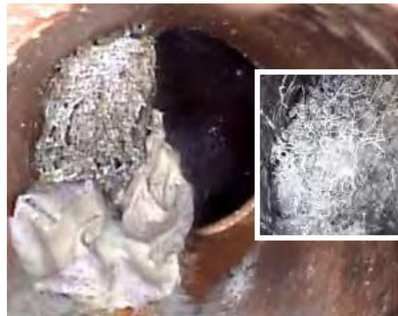
Clay pipe root intrusion
