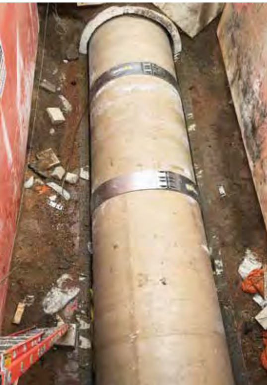
Closure couplings joined both sections of pipe once sliplining was completed in both directions
