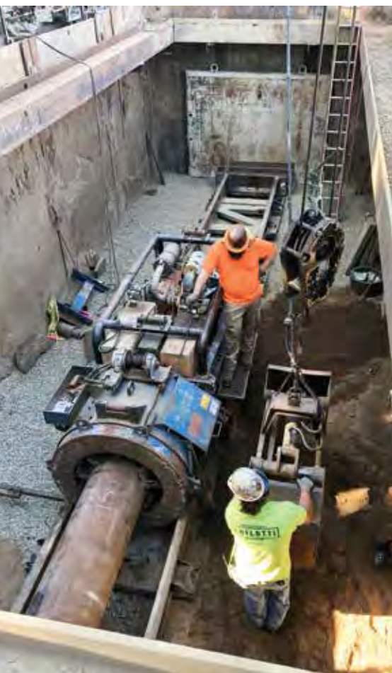
Figure 6. Auger boring installation of 20-inch casing beneath two sets of UPRR tracks.
