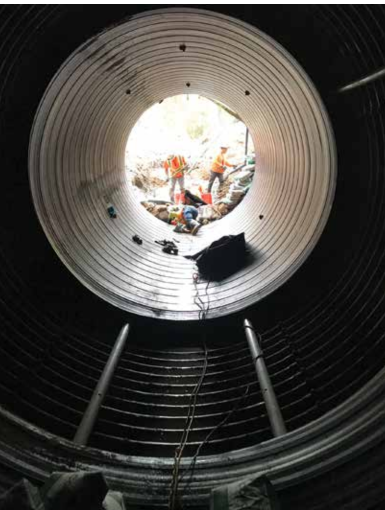
Guide rails ensured proper liner pipe alignment and elevation while decreasing friction during installation
