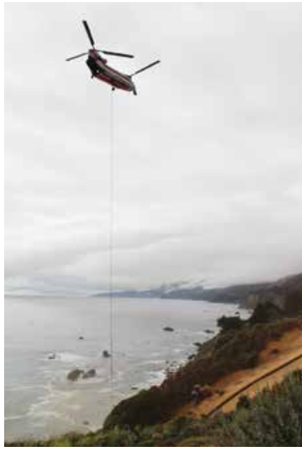
A Chinook helicopter was used to hoist the two tunnel machine sections. The heaviest pick was just under 25,000-lbs.
