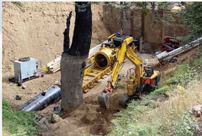
Thrust wall was capable of withstanding an ultimate load of 484-tons
