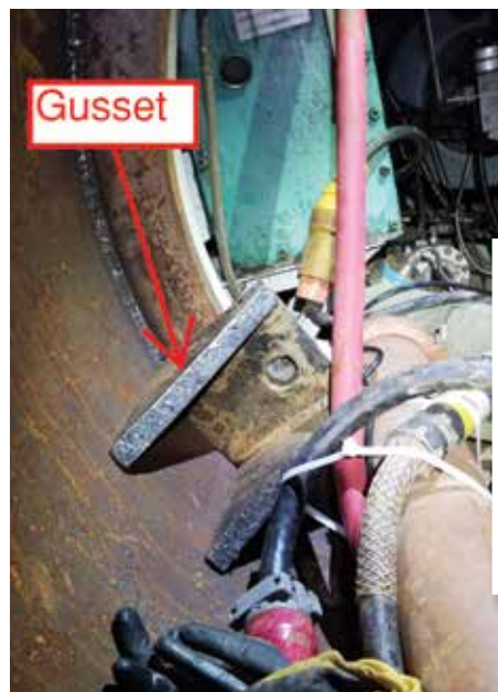
Figure 6. Gusset plates welded to the adapter ring (left); and 1.5-inch gap between the MTBM and the first casing (right)
