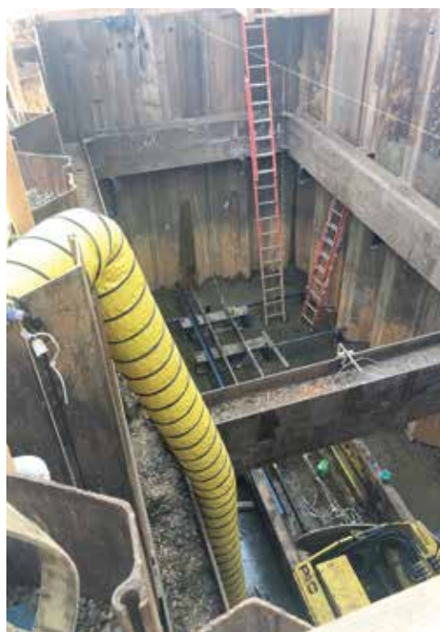
Figure 2. Left: Jacking shaft at Freeway Drive Crossing. Right: Jacking shaft at Highway 29 Crossing
