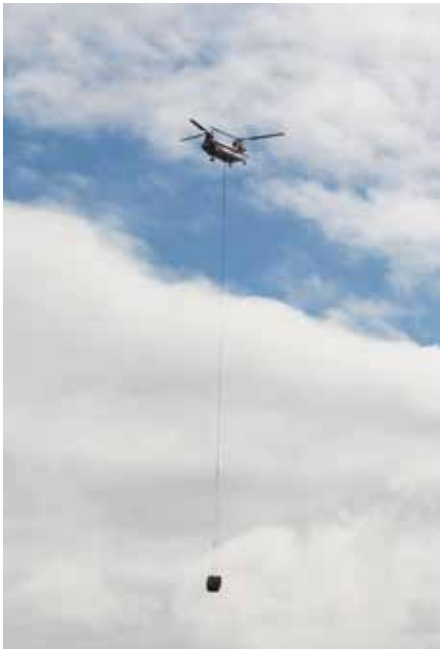
A Chinook helicopter was used to hoist the two tunnel machine sections. The heaviest pick was just under 25,000-lbs.
