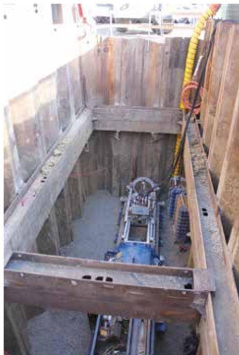
Figure 2. Left: Jacking shaft at Freeway Drive Crossing. Right: Jacking shaft at Highway 29 Crossing
