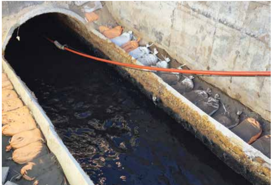
Cleaning of 72-Inch Sewer
