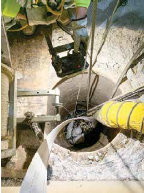
Figure 3. Installation equipment fits through existing manholes
