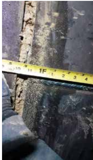
Figure 7. Gaps between casings 5 and 6 (left) and brackets welded between casings 7 and 8 (right)
