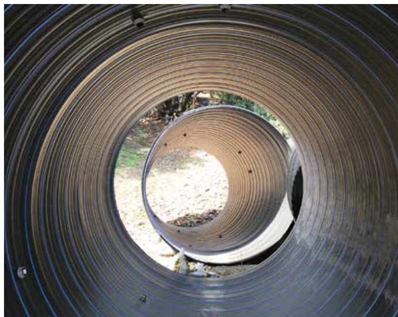
20-foot sections with pre-installed grout ports were shipped from the Ogden UT factory
