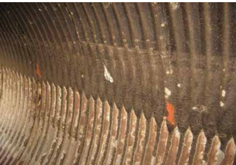
Figure 6. Existing CMP material showing bitumen, zinc, and rivets
