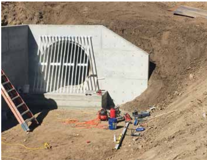
Figure 8. New RCP pipe, headwall, and trash grate before restoration
