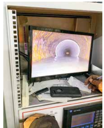
Figure 2. Heavy tuberculation was removed with chain cutters
