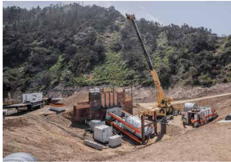
Additional soldier piles were installed at the front of the pit to pin the 800-ton capacity jacking frame back, preventing it from sliding forward as the rams were retracted
