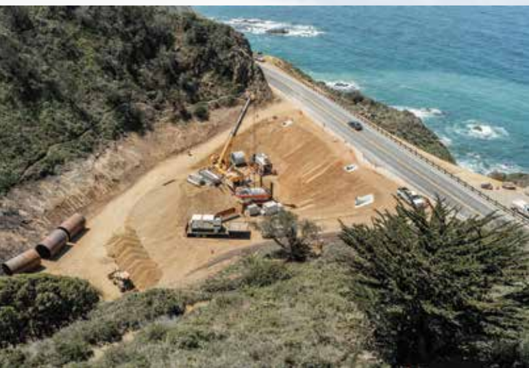
Slope was designed at 30.56 percent downhill which is nearly 80-feet of fall over the 250-foot drive. The culvert was a 1-inch wall steel casing in 16-foot lengths
