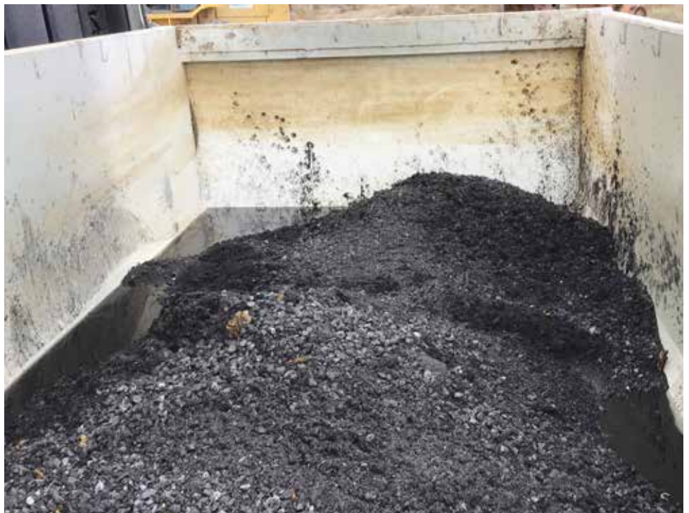
Debris cleaned from sewer. 1202 tons of material was removed!
