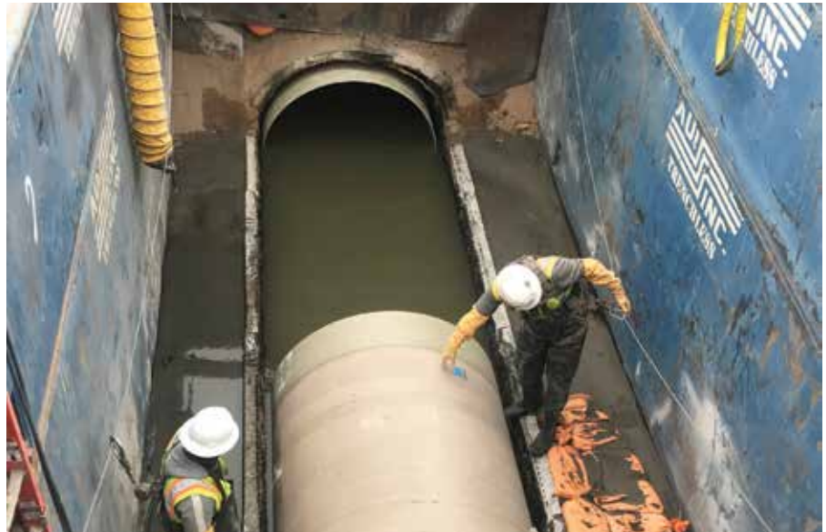
Cleaning of 72-Inch Sewer
