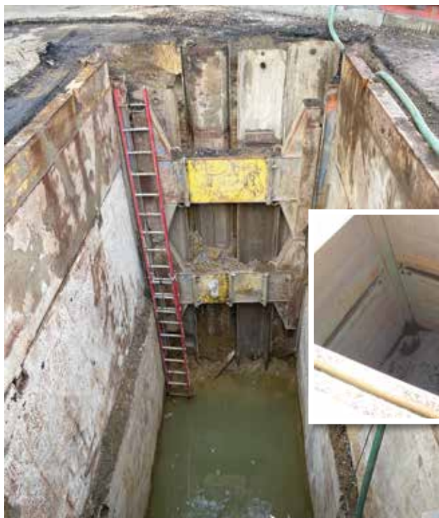
Figure 2. Left: Jacking shaft at Highway 29 Crossing Right: Jacking shaft at Freeway Drive Crossing
