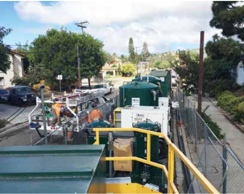
Figure 2. Onsite GAC treatment plant
