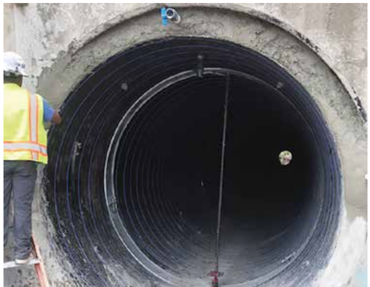
The entire length of the 326 LF culvert was lined with DuroMaxx SRPE liner pipe, providing a long-lasting structural solution
