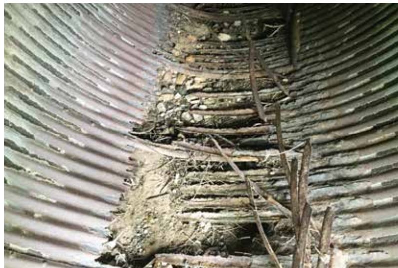
Figure 7. Failed CMP invert before being cast with concrete
