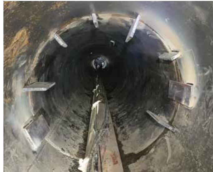
Figure 7. Gaps between casings 5 and 6 (left) and brackets welded between casings 7 and 8 (right)
