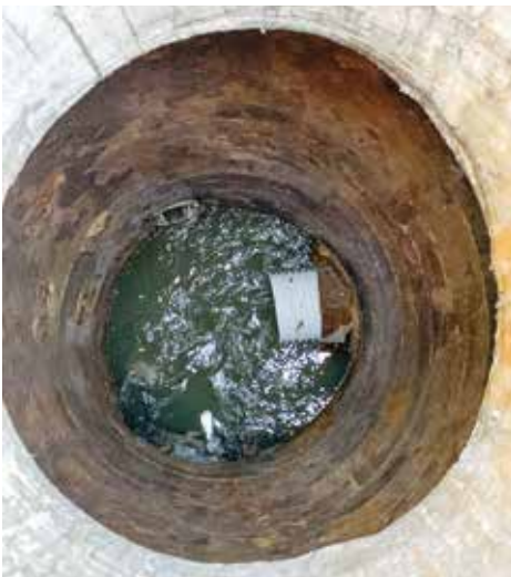
Figure 4. Over 300 linear feet were lined using SPR™EX
