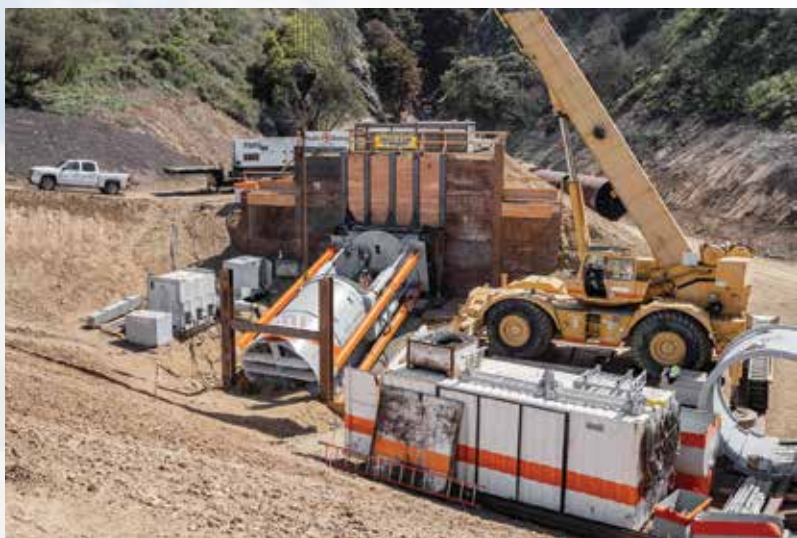
Because the tunnel started inside a depressed basin, there was no jacking pit excavated
