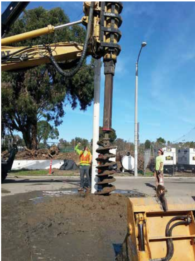
Figure 4. Over 250 wells were drilled at depths ranging from 35 to 40 feet
