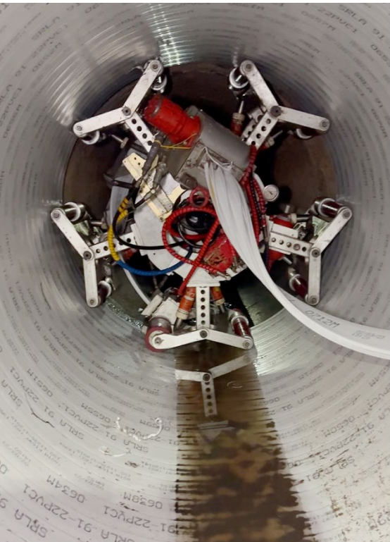
Spiral winding machine “lays” PVC liner directly against host pipe wall
