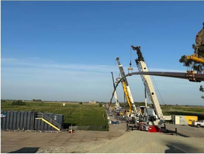
Figure 10. 16-inch gas pipeline supported by cranes during pullback
