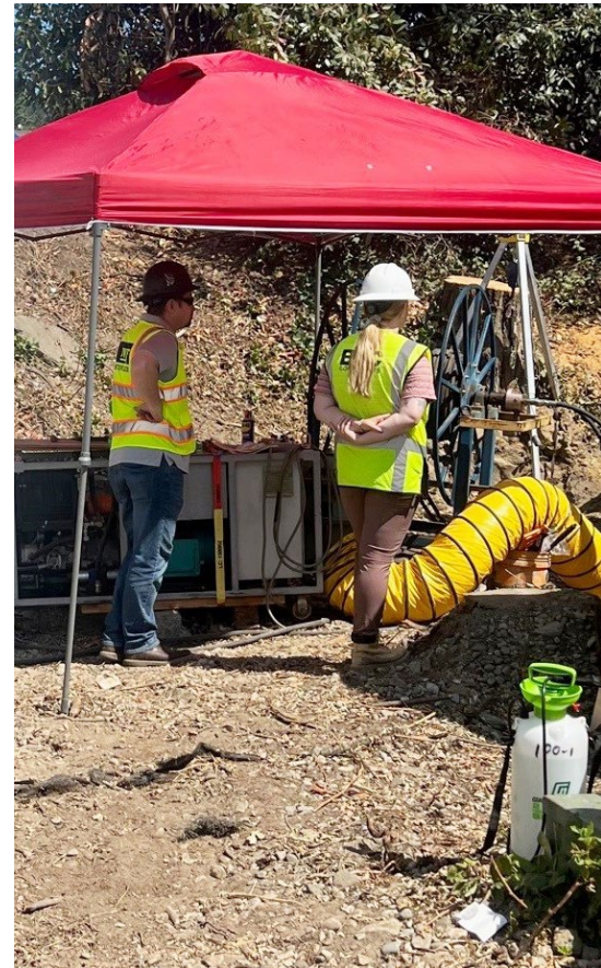
Trenchless pipe rehabilitation method has minimal construction footprint
