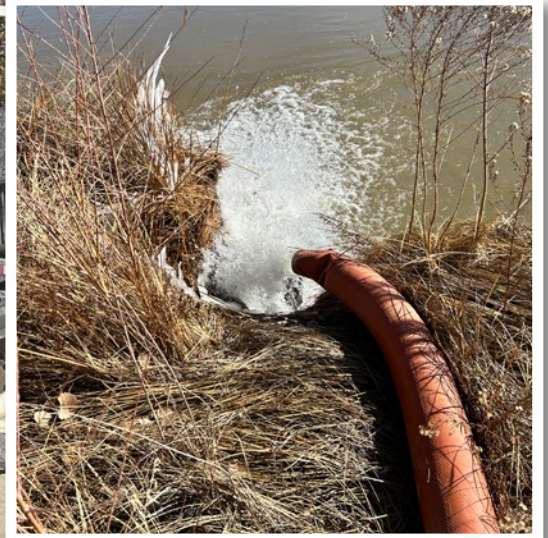
Dewatering groundwater into the Rio Grande
