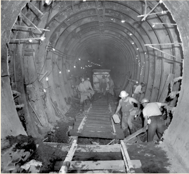
1953 - 12-Foot tunnel preparing for next segment by removing tracks
