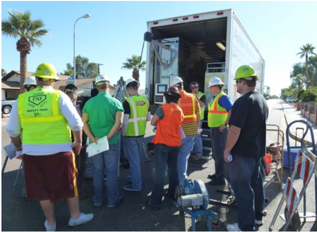
Figure 3. CIPP Site Visit
