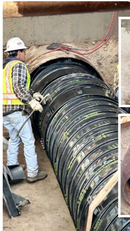
Sliplining 42-inch Ultra Flow Pipe inside 50-Inch Steel Casing
