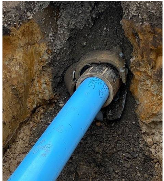
Figure 5. Pipe Bursting Existing 8-inch pipe w/new FPVC
