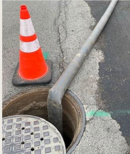
Figure 9. Temporary sewer bypass from manhole to downstream manhole
