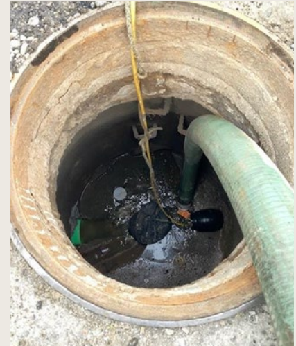
Figure 10. Temporary bypass into manhole
