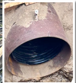
Sliplining 42-inch Ultra Flow Pipe inside 50-Inch Steel Casing
