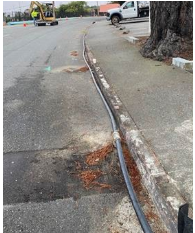
Figure 3. 2-inch HDPE temporary water bypass
