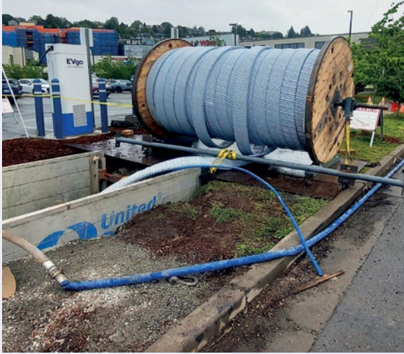
Minimal space required: The reel with the coiled folded liner could be placed next to the electric vehicle charging station
