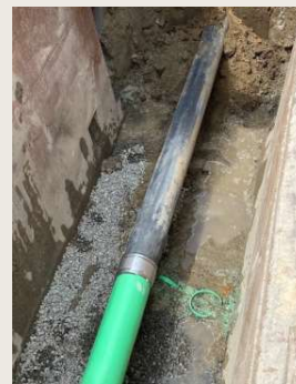
Figure 13. HDPE to PVC sewer main reconnect
