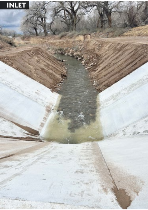
Concrete head walls and rip rap allowed for smooth transitions from earthen channel into new pipe
