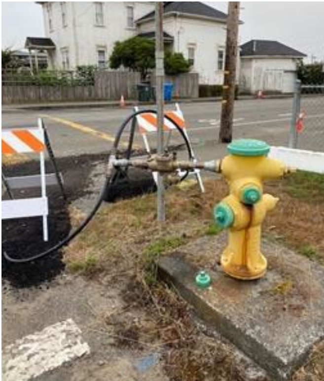
Figure 2. Temporary bypass being supplied from fire hydrant
