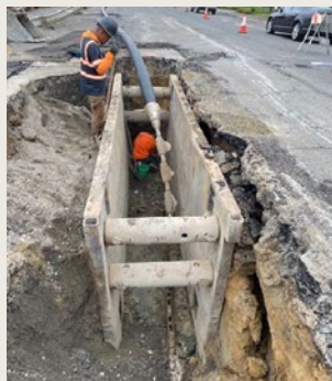
Figure 12. Launch Pit – 8-inch HDPE Sewer Pipe Bursting
