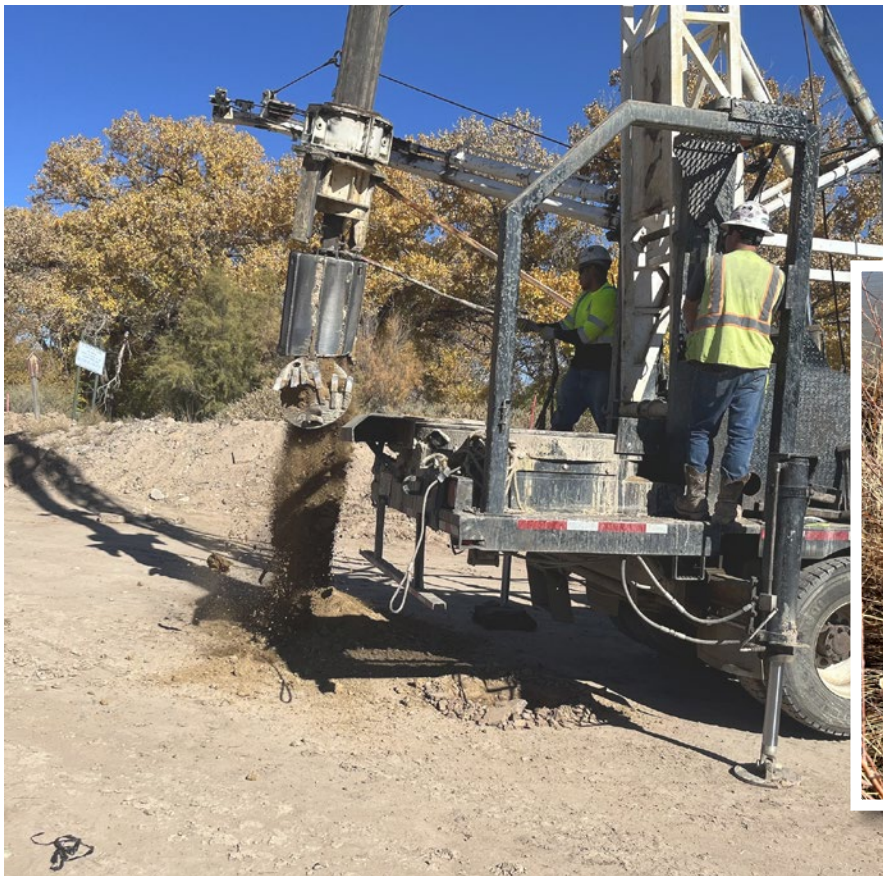
Drilling deep wells for dewatering
