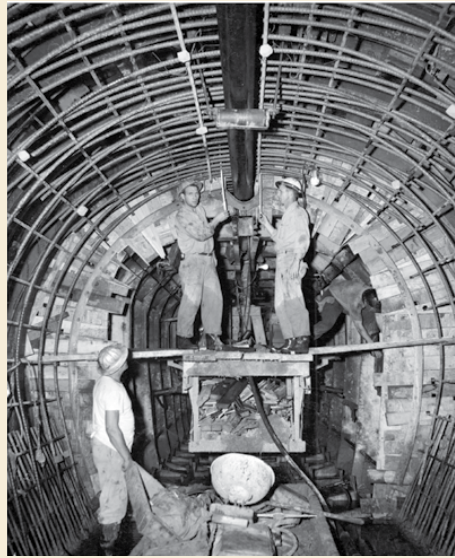
1953 - 12-Foot Tunnel Arch Support Construction
