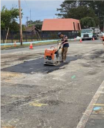
Figure 8. Backfill and Pave access pits each day after pipe bursting
