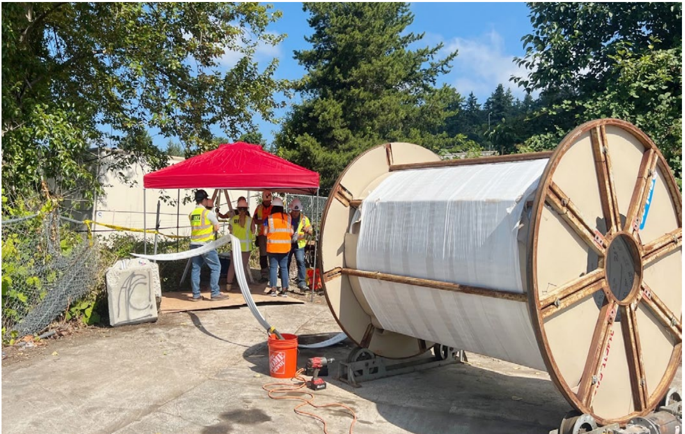
PVC liner is fed from above ground spool
