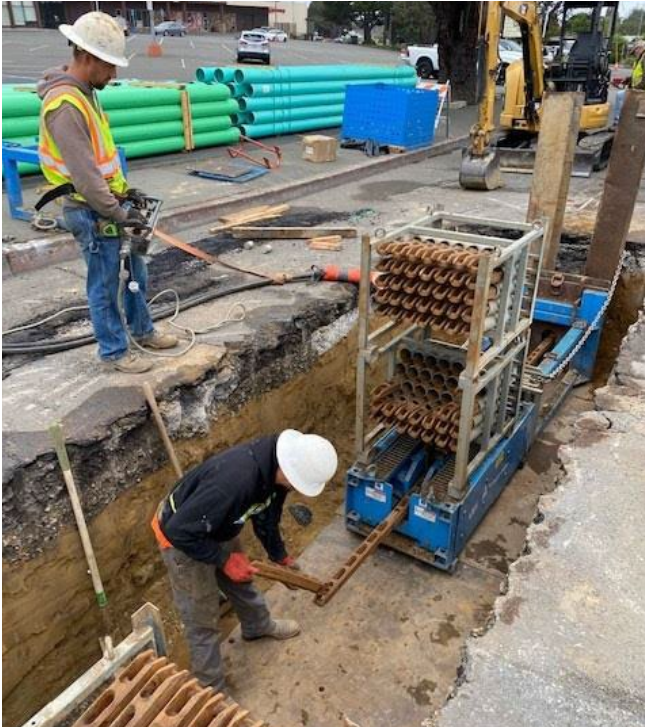
Figure 4. 800G Grundoburst Static Pipe Bursting System
