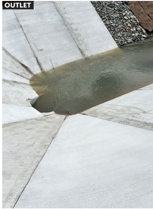
Concrete head walls and rip rap allowed for smooth transitions from earthen channel into new pipe
