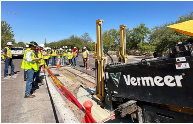
Figure 2. HDD Site Visit
