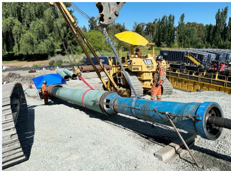
Figure 5. Installing the telescoped conductor casing at the eastern entry point
