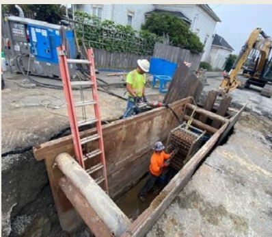
Figure 11. 800G Grundoburst Static Pipe Bursting system and crew for sewer
