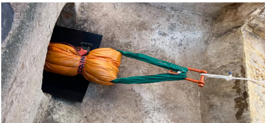
Liner pulled through to vault, ready for inflation
