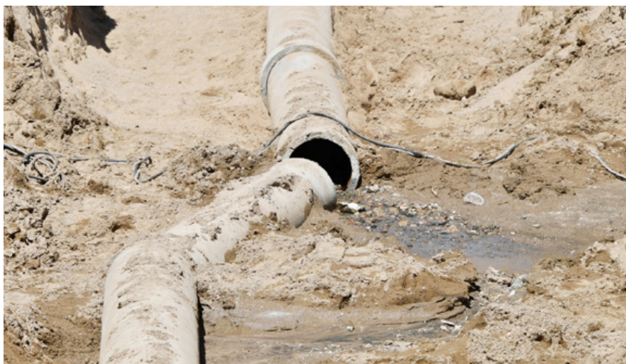
RIDGECREST, Calif. - A formerly straight section of pipe broken by shifting earth during a 7.1 earthquake that shook Southern California in July 2019, cracking buildings, breaking roads and causing power outages. The quake, centered 11 miles from the Ridgecrest area, is the largest quake to hit Southern California in at least 20 years. It was followed by a series of large and small aftershocks, including a handful above magnitude 5.0. (Credit: Gene Blevins/ZUMA Wire/Alamy Live News)
