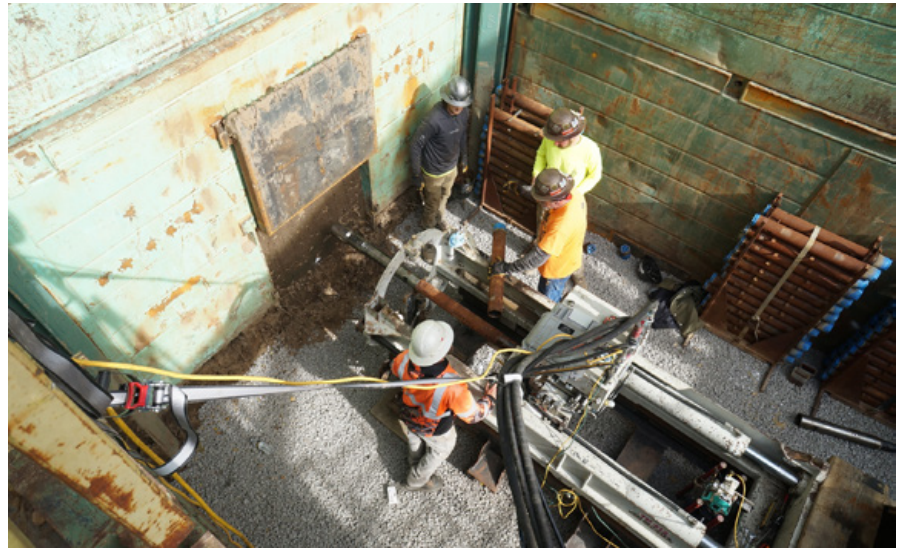
Figure 4: Launch of the pilot tube
