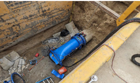
Installation requires only two small access pits
