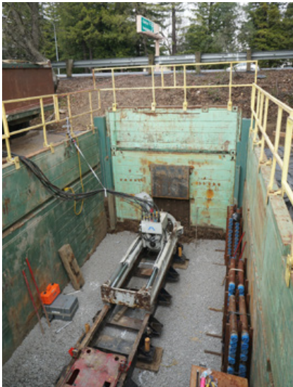
Figure 3: Final configuration of the jacking pit
