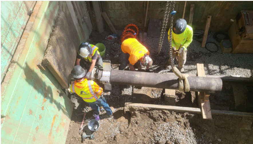
Figure 6: Installation of the ductile iron carrier pipe
