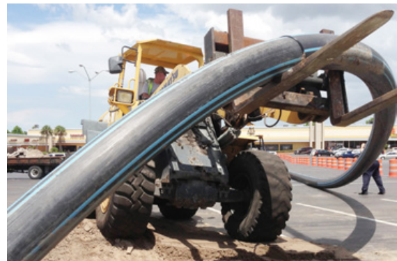
The ductility of HDPE pipe provides high resistance to earthquakes and is also an important factor for ease of installation
