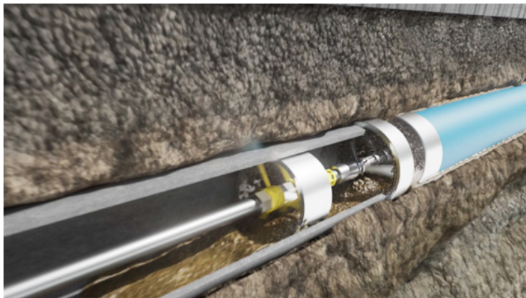
Figure 3. Grinding of AC pipe and mixture with drill mud creates the slurrification during the process
