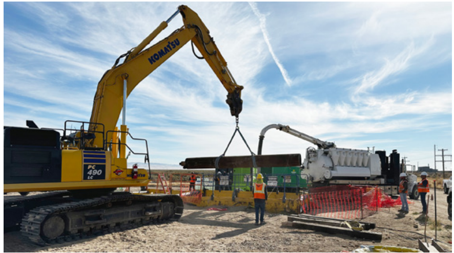
Horizontal Down-Hole Hammer Boring is a trenchless method for new installations
