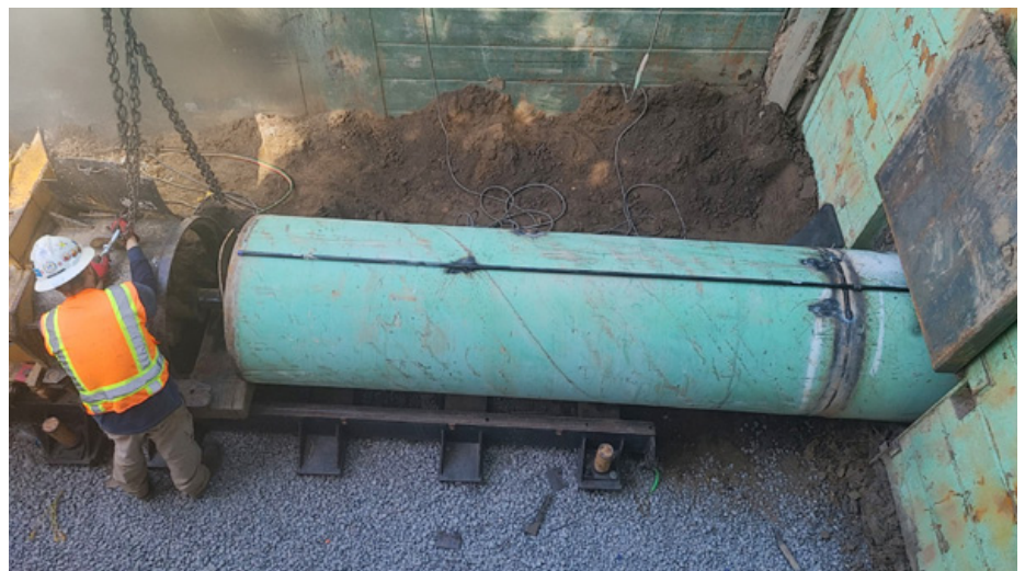
Figure 5: casing installation showing 1/2-inch lubrication pipe
