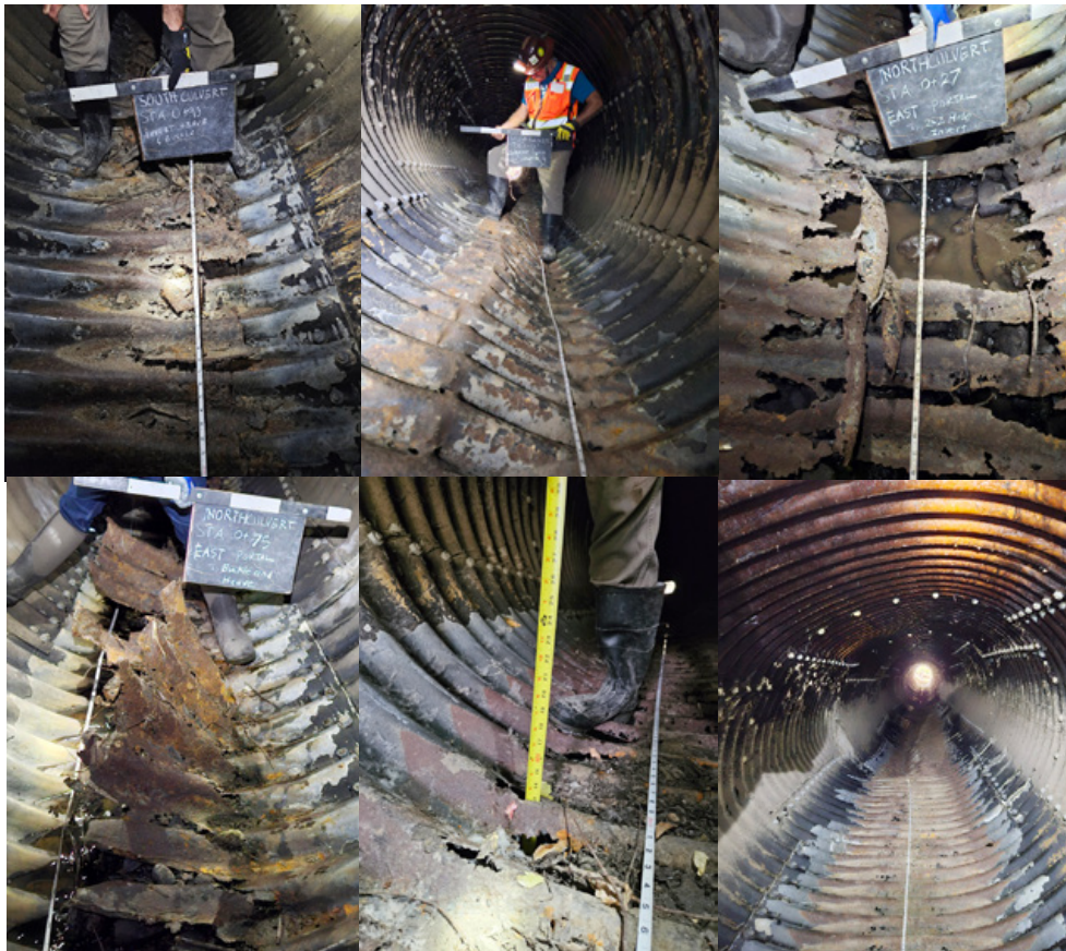
Figure 4-1: Invert condition photos showing a) overlap, b) buckling and heave, c) corroded holes, d) protrusions, e) voids up to 13" deep, f) sag
