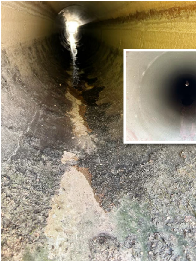
24-Inch Raw Water Main before (left) and after 24-Inch UV CIPP (above right)
