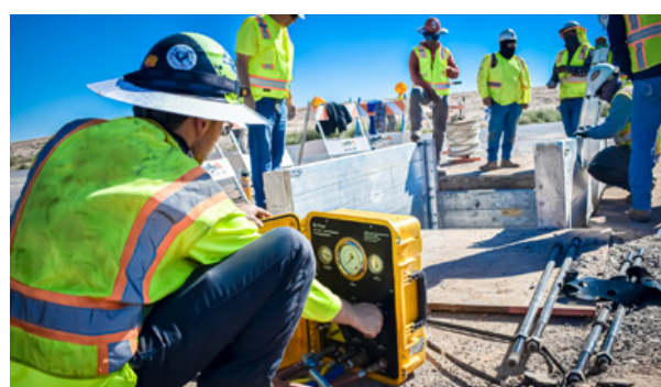
BulletLiner™ has a basic three step installation procedure: 1) fold the liner into a U-shape, 2) Pull the liner through the host pipe, and 3) expand the liner
