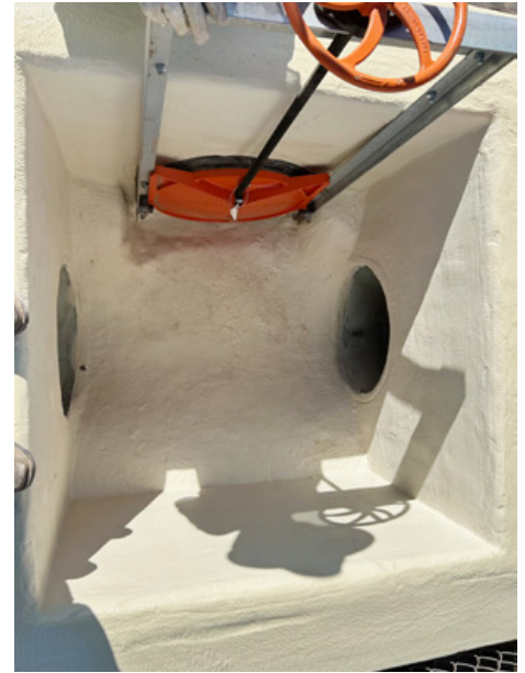
Vault rehabilitated with Zebtron coating
