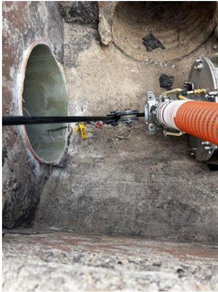
Liner inflated and readied for curing with the light train
